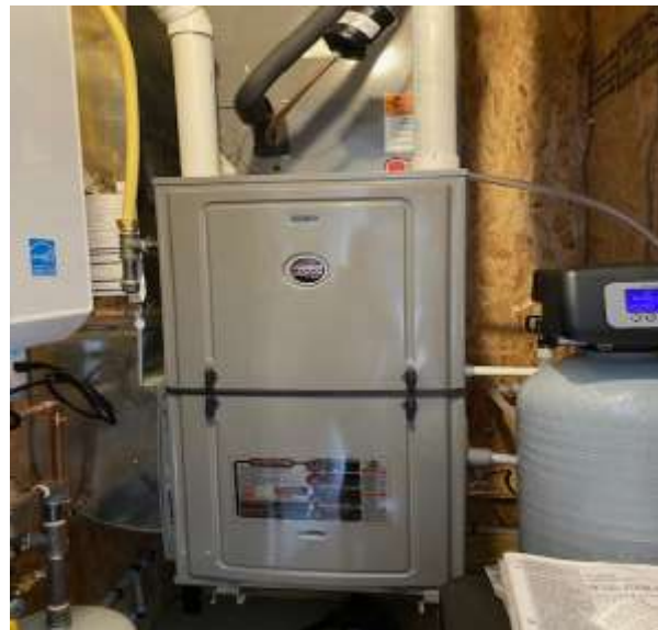
Furnace with Air Conditioner Indoor Coil
